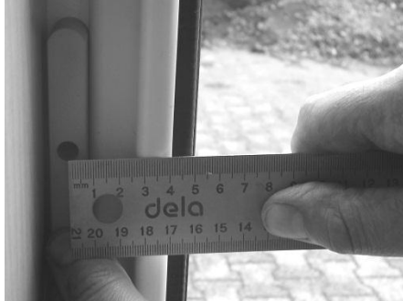
1 – Measure dimension A (in this case 50 mm)
