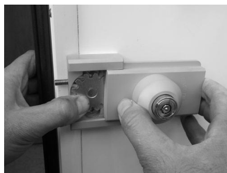
9 – Fit slider and lightly tighten M6 short screws
