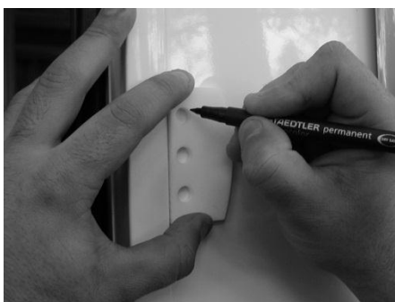
5 – Mark and drill 3 x Ø 9 mm holes
